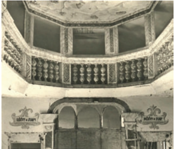
Fig. 32: View of pulpit and women's gallery after dismantling the wooden furniture in the Conegliano Veneto synagogue (U. Nahon Museum of Italian Jewish Art pictures Archive Collection)
